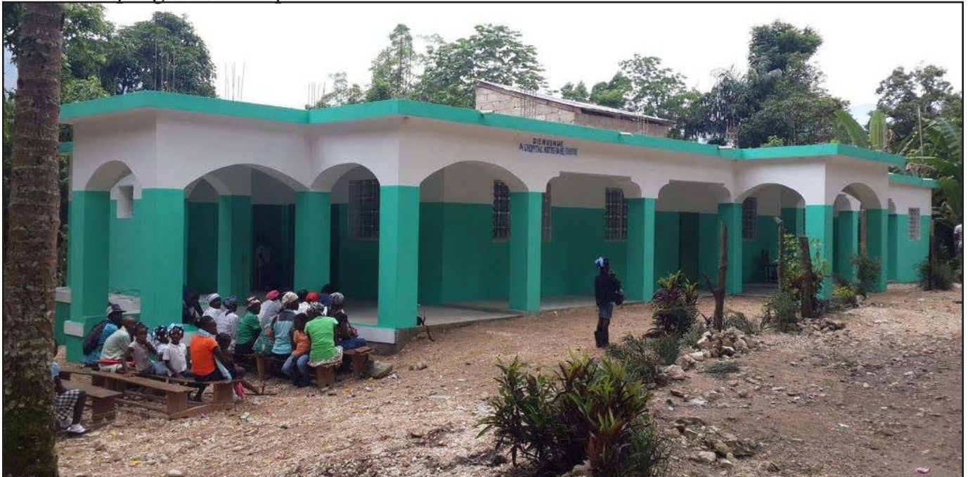
The new health clinic in the village of Chauffard was built with the help of your support! The previous clinic building was 60 years old and damaged in the 2010 earthquake.
